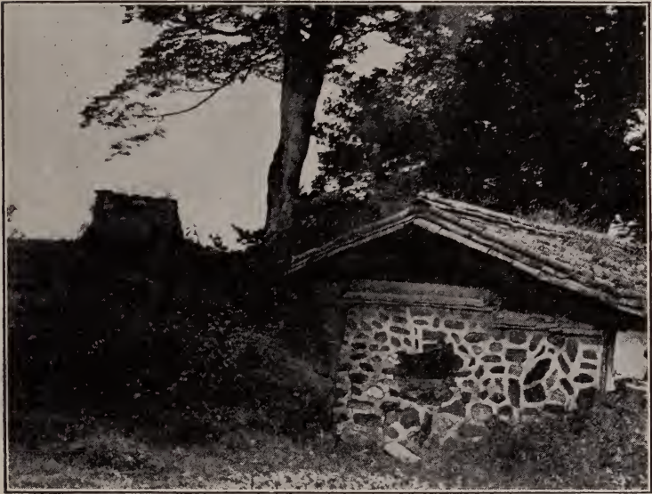
BEACON TOWER ON NAM SAN
